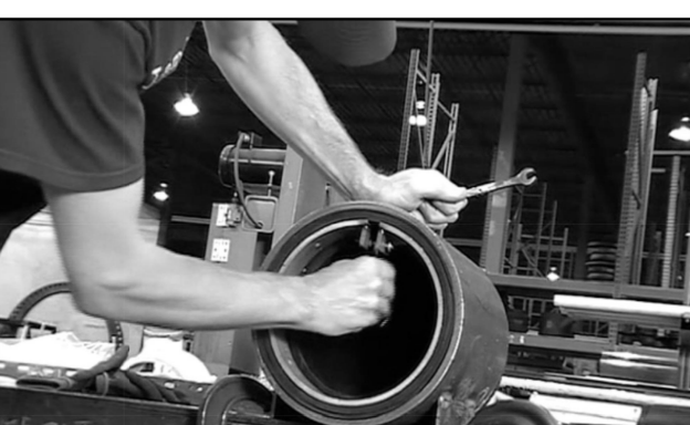
STEP F: Once in place, tighten the clamp to secure it against the pipe and compress the rubber adhesive strip.
